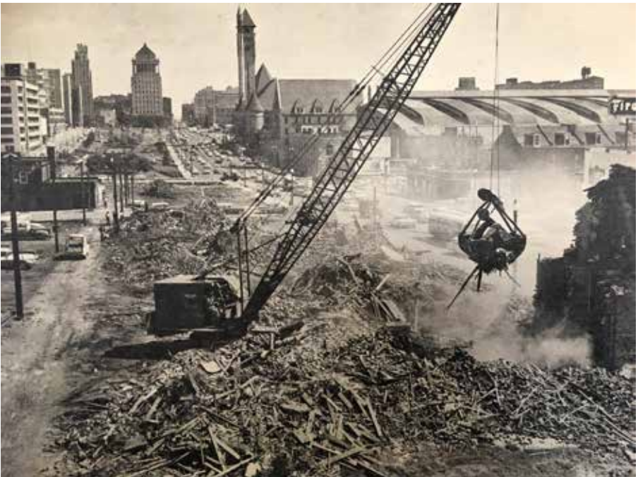
Demolition begins in the Mill Creek Valley. Source: St. Louis Globe-Democrat , 1959.
